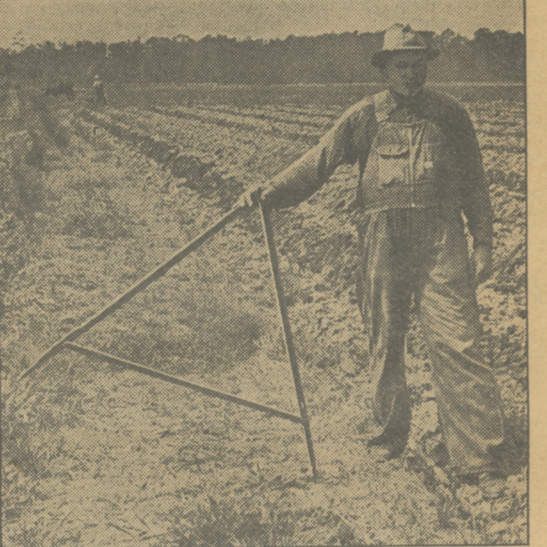
A mathematical agricultural crisis hit Hyde county, N. C., along with the federal government's crop allotments. Community farmers have been used to measuring their land in units of corn hills with a triangular "corn fork," as shown in the picture. In studying federal regulations, many farmers just can't make acres (roughly equivalent to between 2500 and 2750 hills of corn) jibe with their traditional practice.
