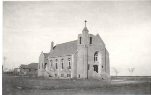
Fig. 25 Photograph, completed St. Mary's structure, circa 1929
