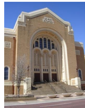
Fig. 49 Photo of First Baptist Church, Amarillo, Texas
